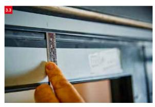
Ensure that there is a 12mm gap top and bottom between the outer frame and the door panel.
