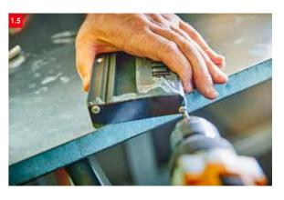
Fit the end cap. Note! This is not just an aesthetic piece. It must span the full depth of the subcill as it acts as a physical barrier to stop water ingress.
