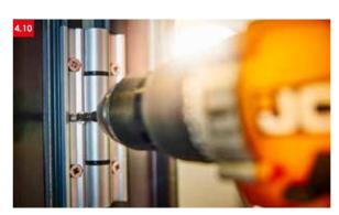
Important! Once the door is operating correctly and the 12mm gap top and bottom has been maintained, lock off by fitting 4.2 x 25mm stainless steel countersunk self tapping screw to rollers, guides and hinge. If the frame and doors arrive as an assembled unit check to see if these locking screws have been fitted in the factory.
