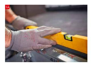
Place the subcill on to the substrate and level the subcill, if necessary using packers. Laser levels are ideal to assist with this process, particularly on wide installations.
