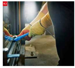
Position 2 packers, one inline at the corner that is to be toe and heeled with the other at 90° on the opposite side.
