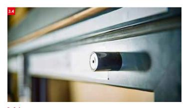
3.4 Check that the traffic door magnets have been fitted and that they align when in the open position.
